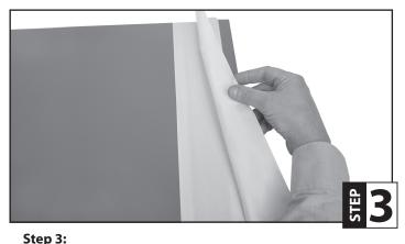
Be sure to unfold the film, extending it 3" from the foam.
